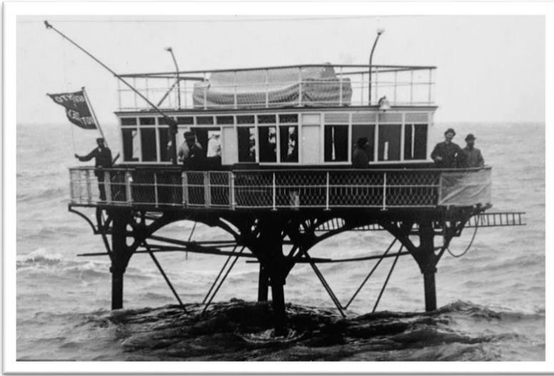
The rails were submerged in all but the lowest tides but the trolley car stood 23 feet high above the track, supported on four legs which each sported four wheels. The two-tier car featured an ornate saloon, complete with potted plants and a refreshment counter. From there a staircase led to a promenade deck, the better to enjoy the healthy sea air.
